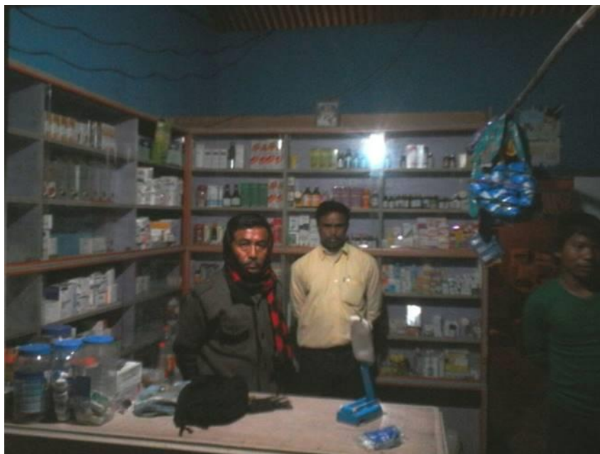
Figure 9: Solar Light Fixtures at Shops
