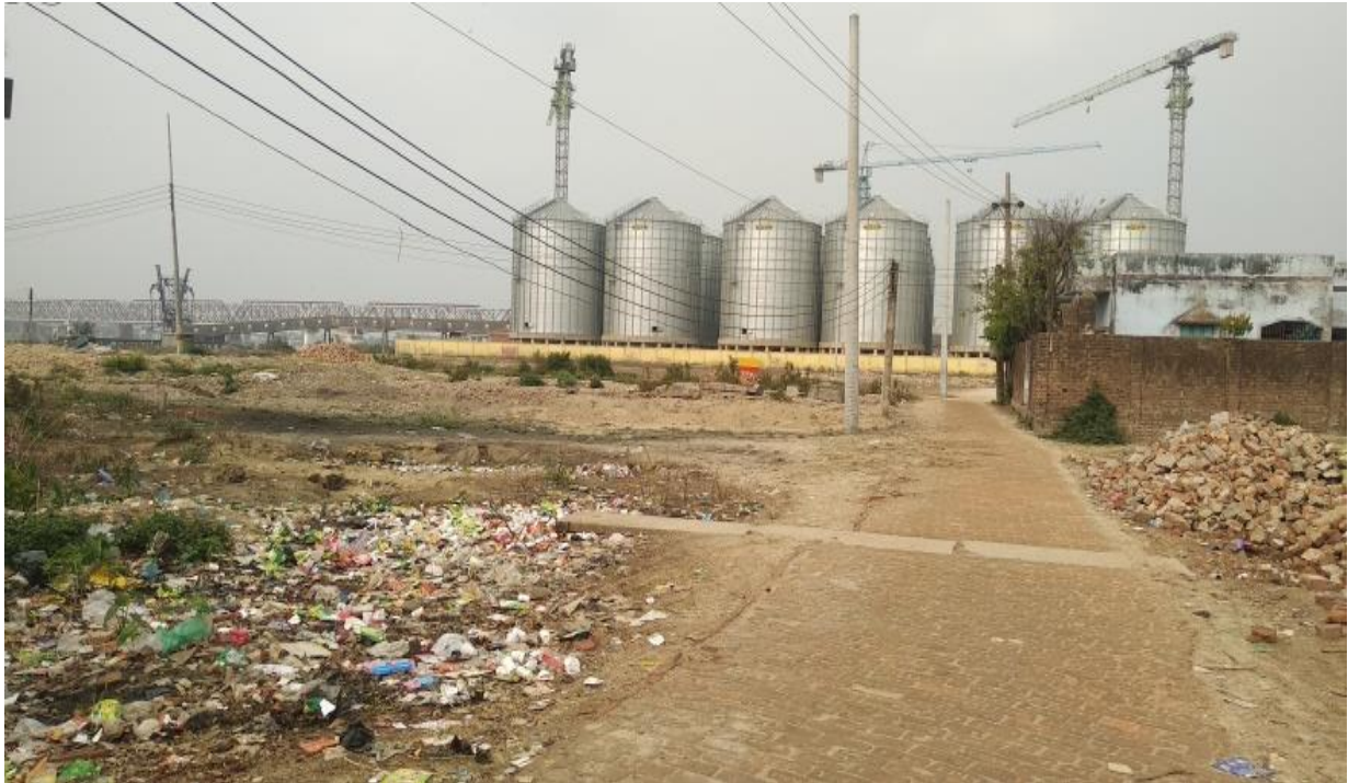
Silos near upcoming ICT
