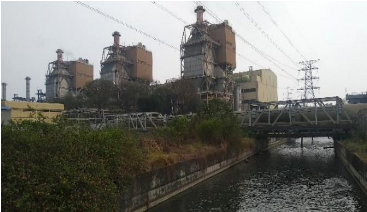
Ashuganj Power Plant and Station
