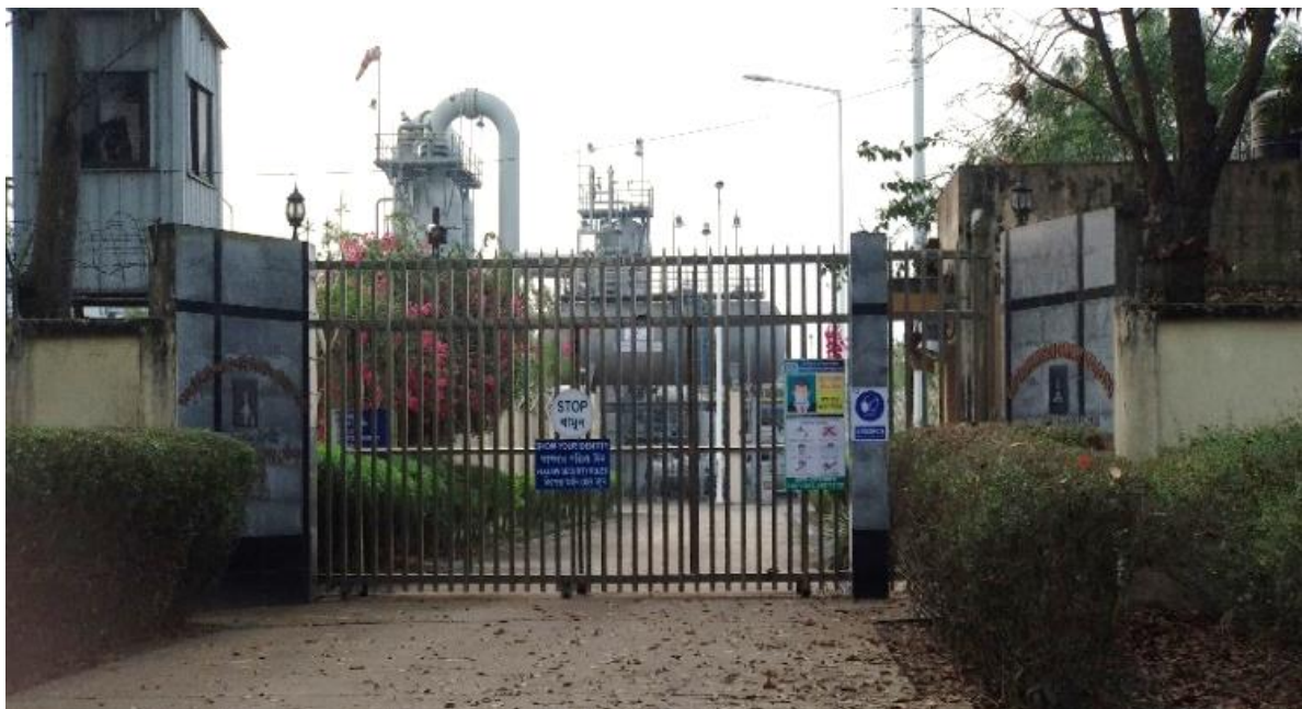
Gas Transmission Company Limited near Ashuganj Port
