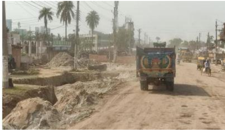
Roads under construction
