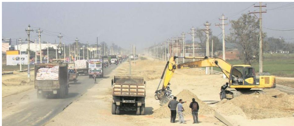
Construction works going on in Birgunj-Pathlaiya Road
