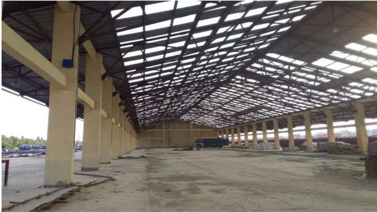
Unwalled Storage Section of Birgunj ICP
