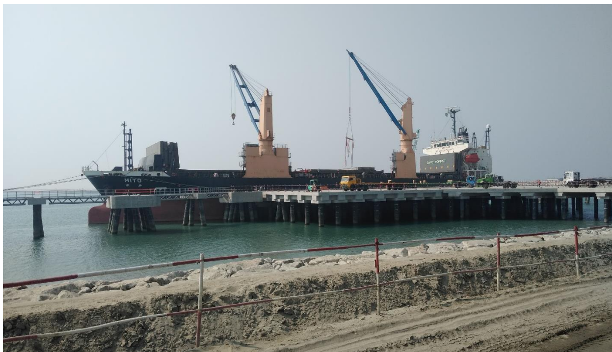
Matarbari Coal Power Plant Jetty
