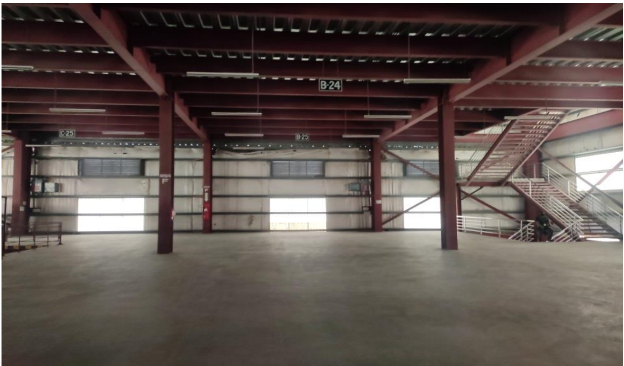
Second floor of the three-storied warehouse
