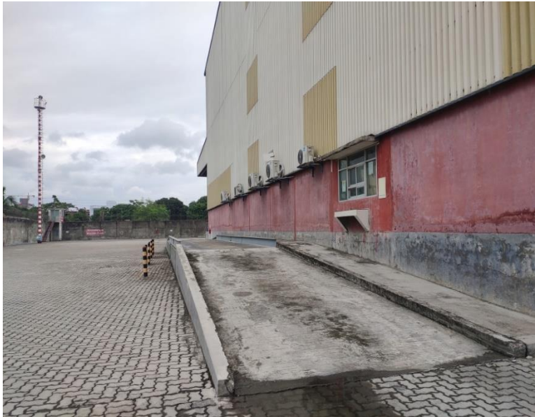
Automated Weighing Station
